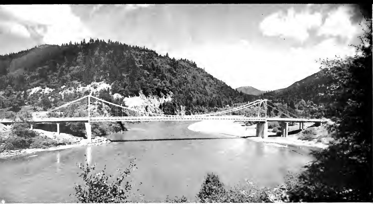
Bridge across Klamath River winner of national award for most beautiful steel bridge costing less than $250,000 built in 1940
